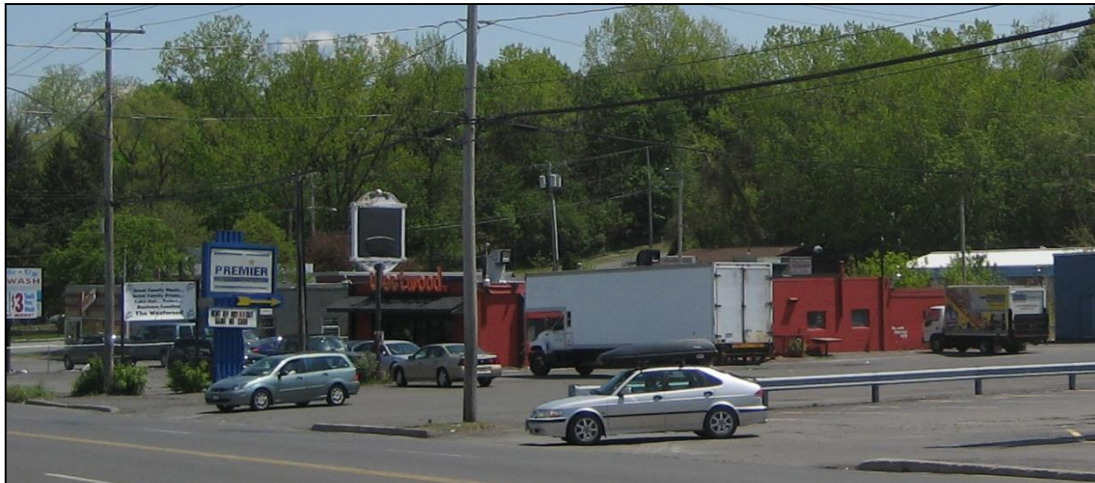
EXISTING CONDITION: Multiple driveways and a lack of sidewalks on the south side of Onondaga Boulevard near the Onondaga / Velasko intersection make for a hazardous and unappealing pedestrian environment.
