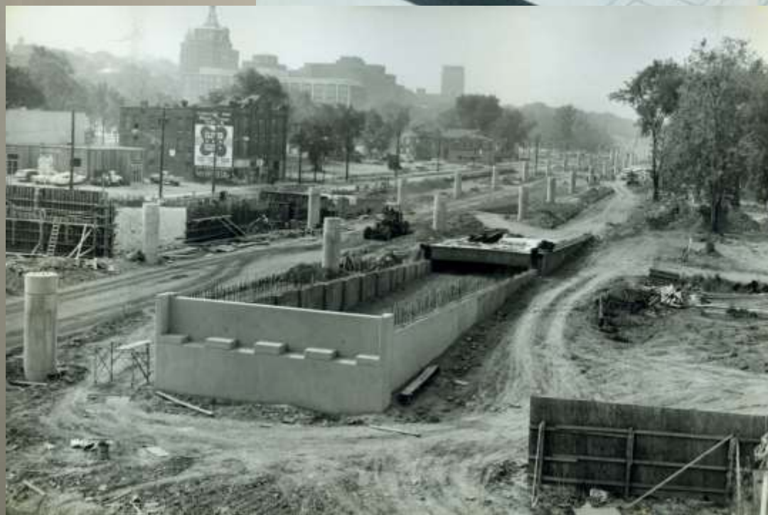
Route 81 Construction 1960s
