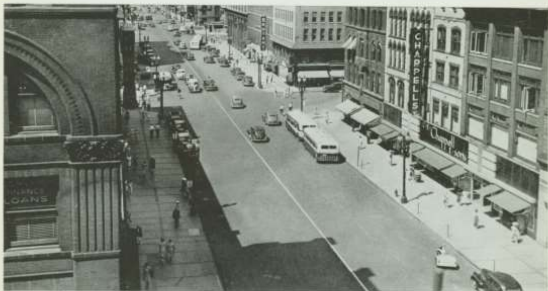
Downtown South Salina street, same view as above, after removal of trolley tracks and repaving. Movement of traffic in the congested downtown area has been greatly facilitated and the business section has undergone a beauty treatment. New buses replacing trolley cars, Salina Street has been thus improved this year from James Street to Onondaga Street. This
